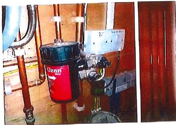
Figure 6 - Exposed pipework within the boiler cupboard.
