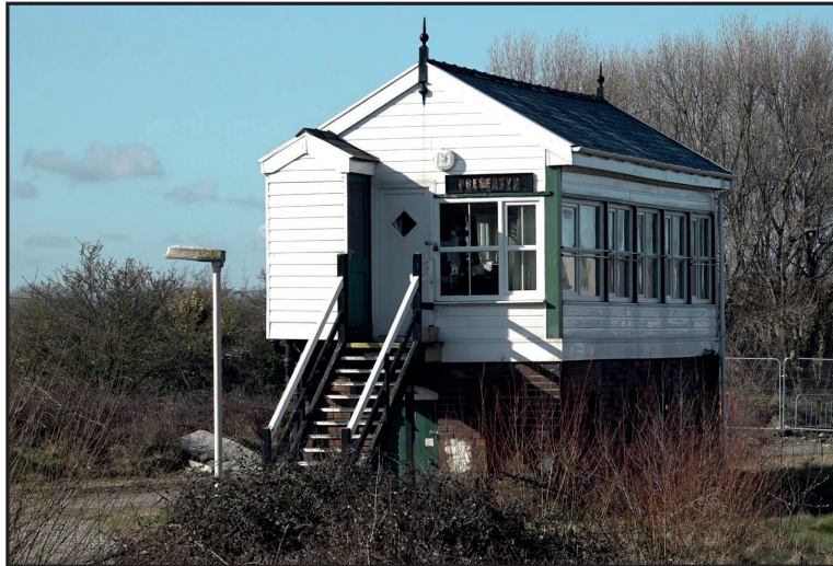
Signal Box immediately before decommissioning in 2018 - Photograph Tony Griffiths
