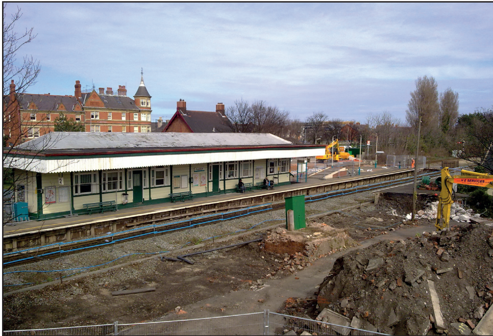
Prestatyn station taken during the installation of ramps and lifts in 2011. Photo Dr James Davies MP
