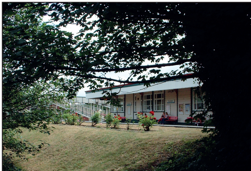
View of the main platform showing the original steps and bridge in the background on the original platform 3
