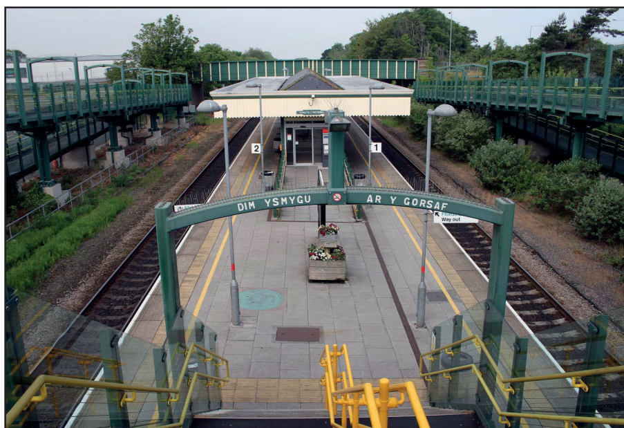
Prestatyn station showing the steps from the bridge onto the main platform and the ramps for people with mobility issues.
