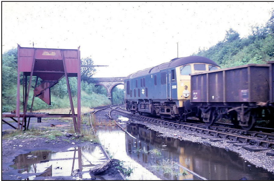
Dyserth station in 1971. Photograph Trefor Thompson
